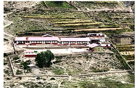
Figure 1 School Building constructed at Namdo of Dolpa
